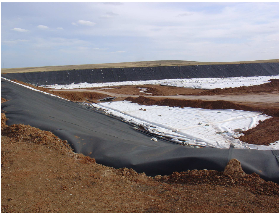
Figure 5. Containment of the landfill cell base.
