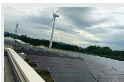
Wind Power Generation at the Fukushima Renewable Energy Institute
