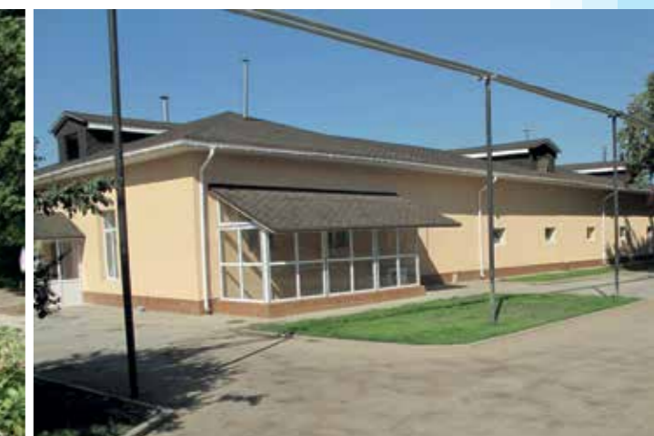
Animal breeding facility main view outside (renovated)
